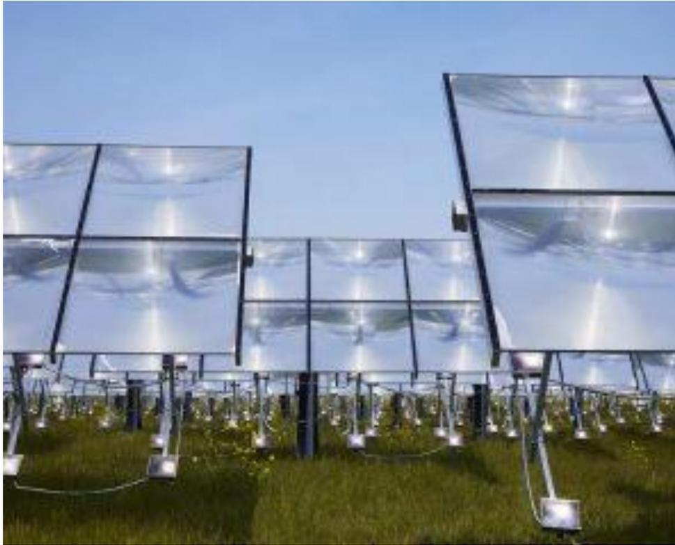
Concentrating collectors (Point Focus Fresnel) deliver heat at around **160 °C** in Hørsholm, Denmark
