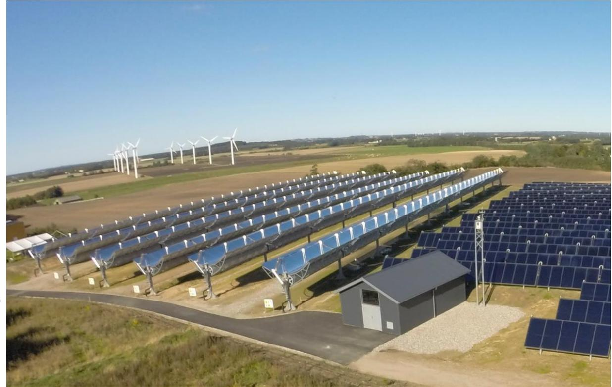
Combination of flat plate collectors (up to 70 °C) and parabolic trough collectors (**up to 95 °C**) in Taars, Denmark
